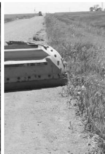
(4) Rear view showing clean recovery of gravel at shoulder.
