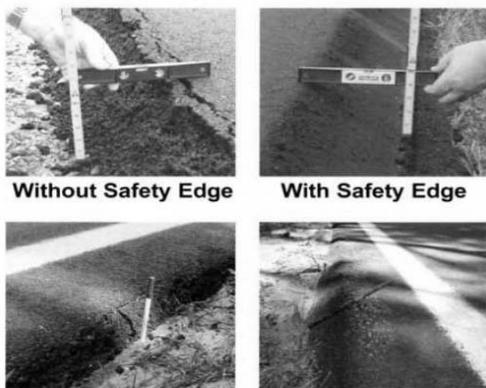
**Figure 3:** For proper edge slope, specify a 30° - 35° angle asphalt fillet "Safety Edge."
