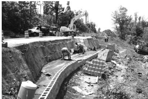
Placing and compacting lightweight sawdust backfill.
